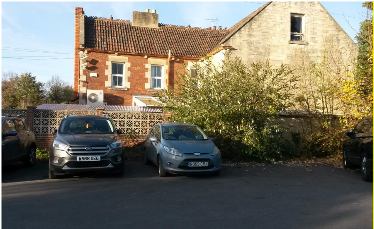
Photo of southern elevation of 17 Polebarn Road from existing car park
